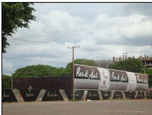
Foto 20: SGCV Lts. 27, 28, 29 e 30 – obra do Park Sul Prime Residence .
